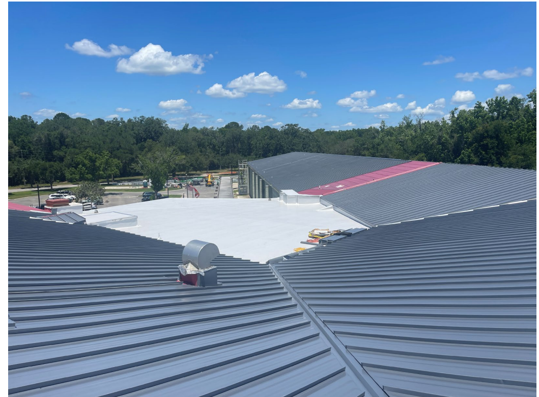
Parrot Phase 1 New Roof
