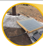
Kelly’s heating system begins with a solar panel on the hogan’s roof.
