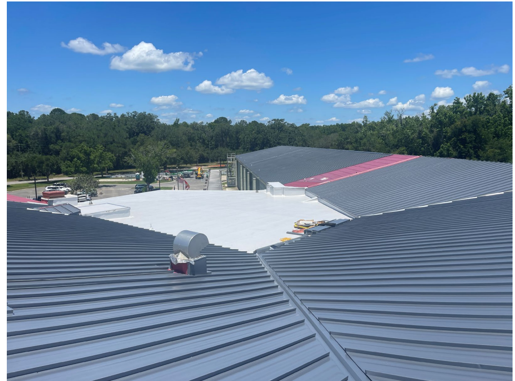
Parrot Phase 1 New Roof
